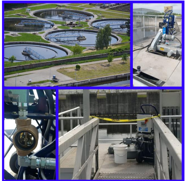
Figure 1: PHoenix on Clarifier Gear
